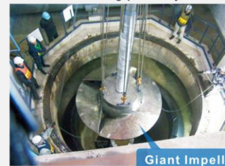
Installation of Large-Scale Drainage Pumps
