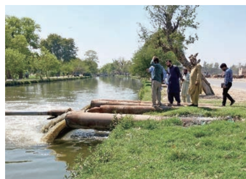
On-Site Pump Drainage Operation
