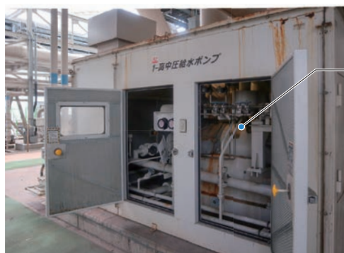
High- and medium-pressure feedwater pump (Boiler feedwater pump)
