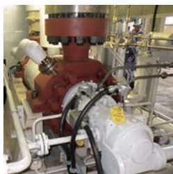
High- and medium-pressure feedwater pump (Boiler feedwater pump)
