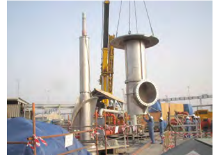
Installation of cooling water pump
