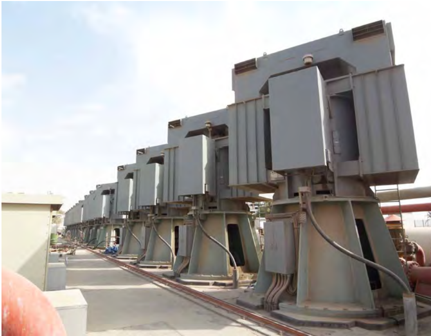
Supply Cooling Water Pumps
