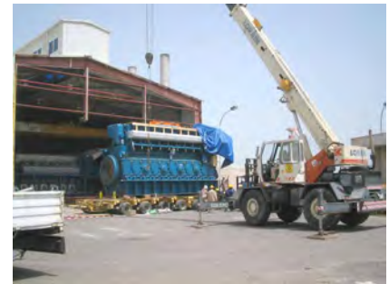
Installation of a 10.5 MVA power generator
