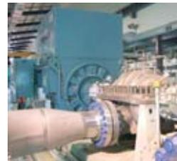
High pressure seawater supply pump (RO)
