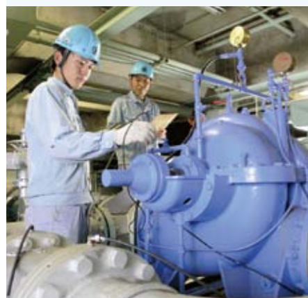
Inspection of pumping equipment
