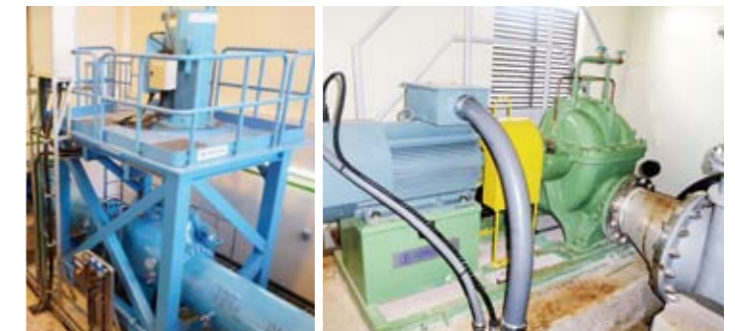
Tuen Mun Water Treatment Works Hong Kong Capacity 76.4m 3 /min Effective Head 19m Maximum power output 211.2kW
