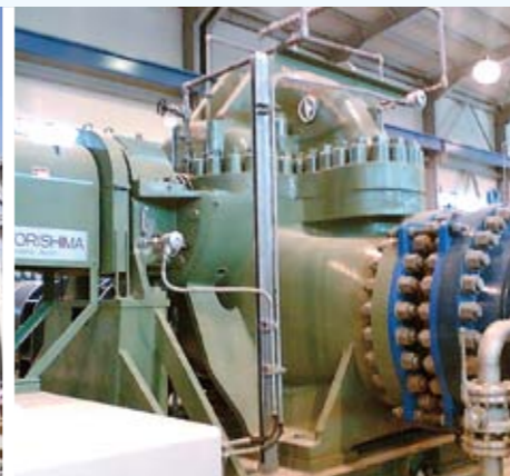
Test and commissioning of transmission pumps
