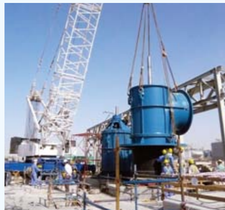
Installation of seawater intake pumps
