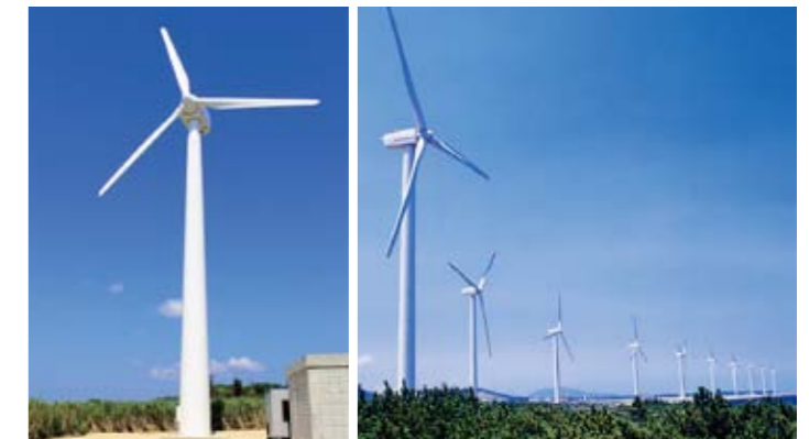
100kW wind turbine
