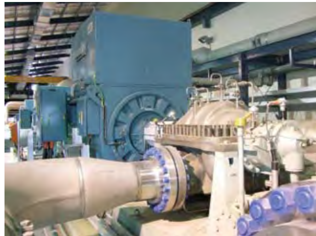
[Horizontal twin-suction axially split multi-stage volute pumps]
