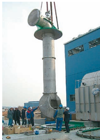
Hot Well Pump for Germencik Geothermal Power Project, Turkey (Size : 1,000mm, Driver : 600kW)
