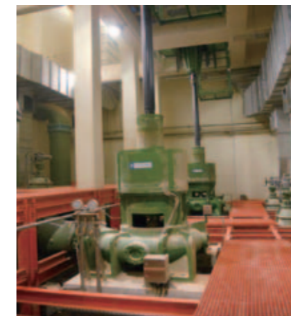
Intermediate sewage pumping station in Dubai, U.A.E.
