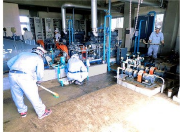
Restoration work at a flooded drainage pumping station after torrential rain
