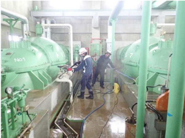
Restoration work at a flooded drainage pumping station after torrential rain
