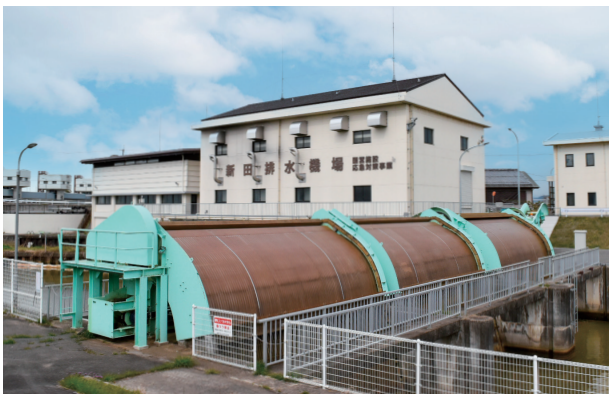
Shinden Drainage Pumping Station
