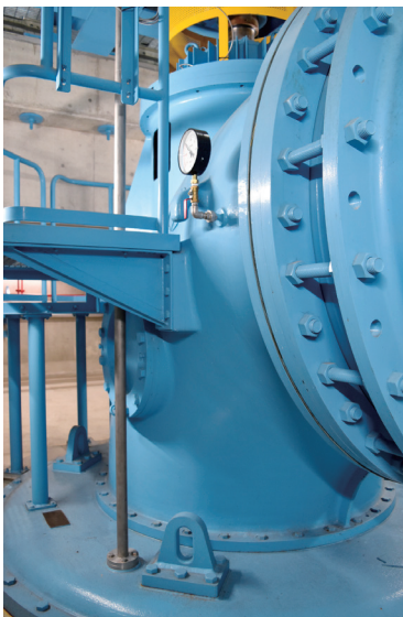
Flood Drainage Pump
