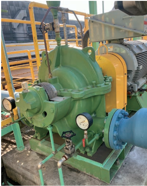
High Pressure Feed Water Pumps for the Rolling System
