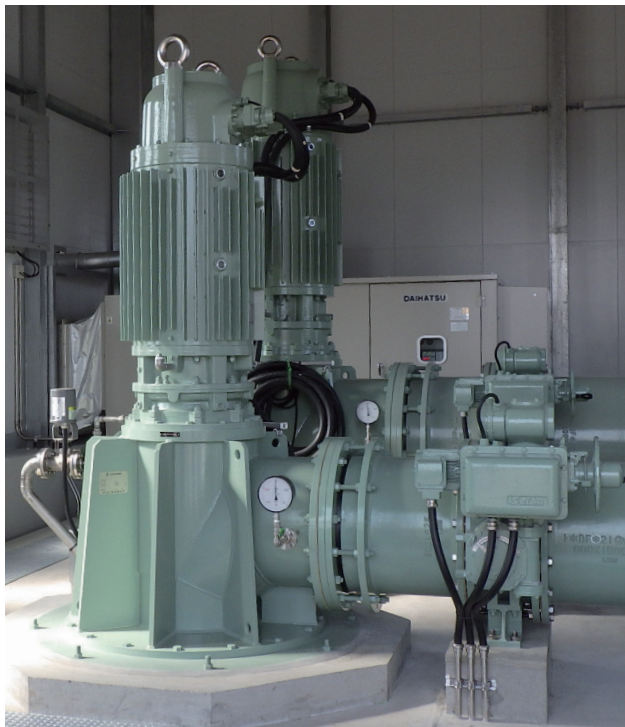
Pump with integrated submersible motor
