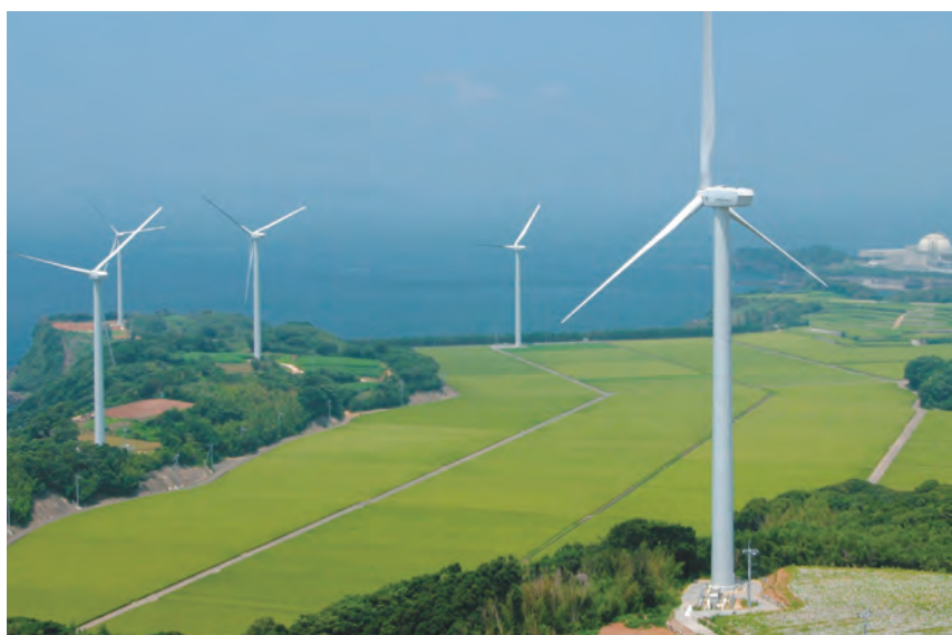
Genkai Wind Energy Development, Genkai Town, Saga Prefecture (1,500 kW × 6 units)
