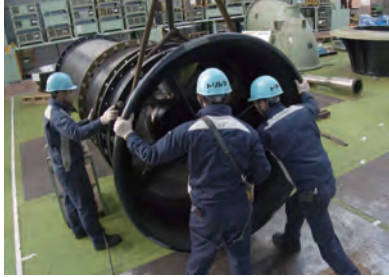
Assembly of large vertical pump
