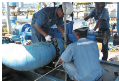
On-site maintenance of pumps
