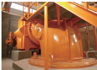
River drainage pumping stations
