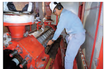
On-site maintenance of pumps
