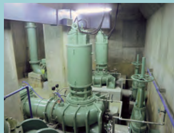
Vertical mixed-flow volute pumps with integrated submersible motor
