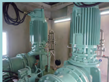
Vertical axial-flow pumps with integrated submersible motor
