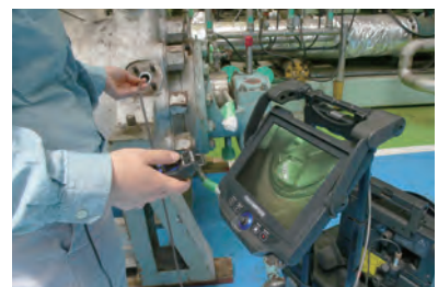
Internal examination of pumps with endoscope camera
