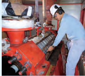
On-site maintenance of pumps
