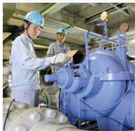
Inspection of pumping equipment
