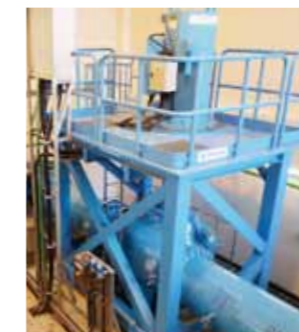
Tuen Mun Water Treatment Works Hong Kong Capacity 76.4m 3 /min Effective Head 19m Maximum power output 211.2kW
