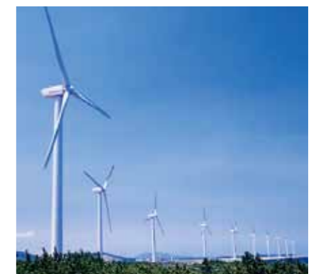
1500kw wind turbine
