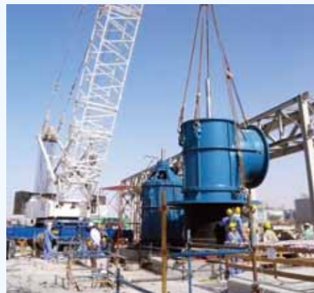
Installation of seawater intake pumps
