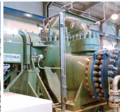
Test and commissioning of transmission pumps
