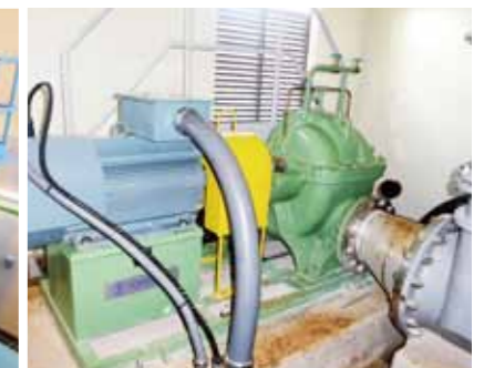
Mukangu Water Treatment Plant2 Kenya Capacity 15.96m 3 /min Effective Head 30m Maximum power output 50kW
