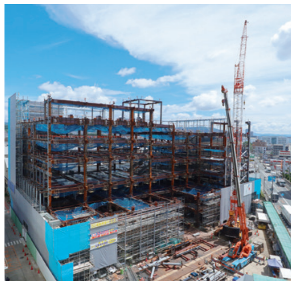
State of construction as of mid-July 2020
