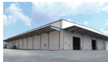
New warehouse for wooden patterns completed in March 2019
