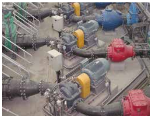
飲料水配水用ポンプ CDM400×350mm, 1,620m 3 /h, 35m, 200kW CDM350×300mm, 1,080m 3 /h, 35m, 150kW
