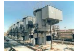
1976 Pumping station for chemical complex in Kuwait
