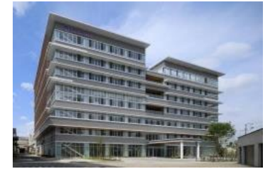
2021 New head office & factory building completed
