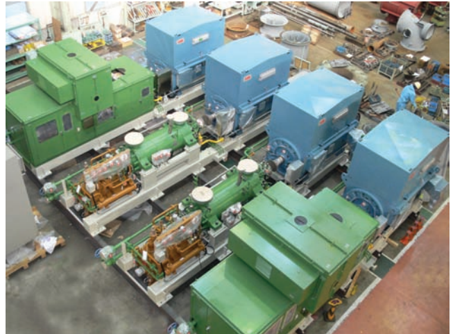
Staythorpe C Combined Cycle Power Plant UK MHG, Boiler feed pump
