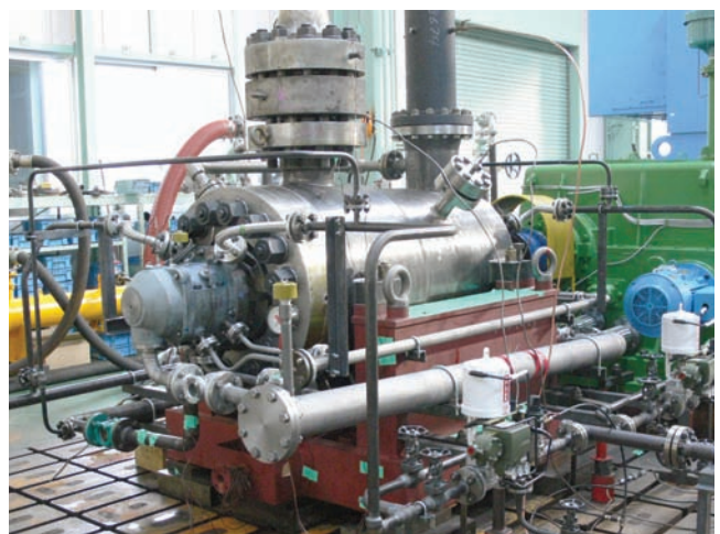
Pacifico Coal Fired Power Plant Mexico MHB, Boiler feed pump
