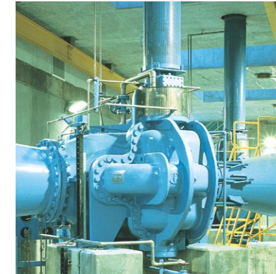
Water distributing pumps Size : 800mm 100m - 111m 3 /min - 2500kW
