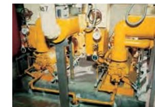
Boiler feed pump for district heating and cooling
