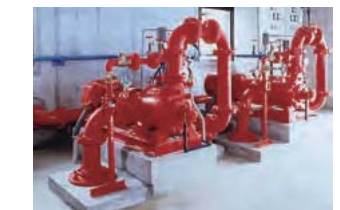
Fire pump for disaster preparedness facilities
