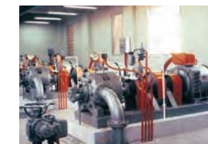
Water transmission pump for potable water facilities
