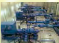
Water transfer pumping station
