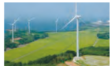
1,500kW wind power generators
