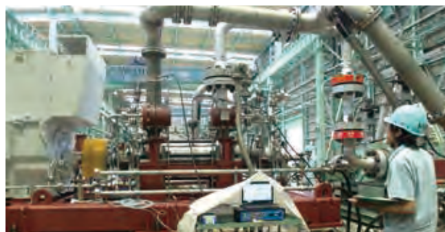
Performance test for a boiler feed pump
