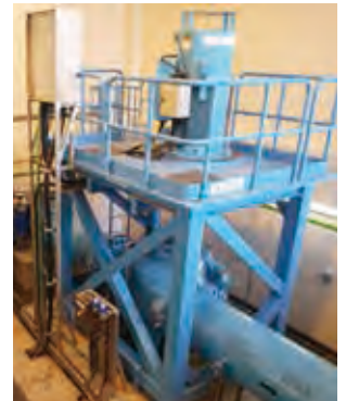
Reverse-rotated pump water turbine installed in Tuen Mun WTW in Hong Kong. This installation handles water flows of up to 76.4m 3 per minute and generates power of up to 211.2kW.
