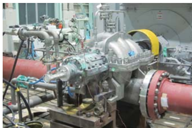
In-house testing of a double-suction centrifugal pump for use in desalination plants
