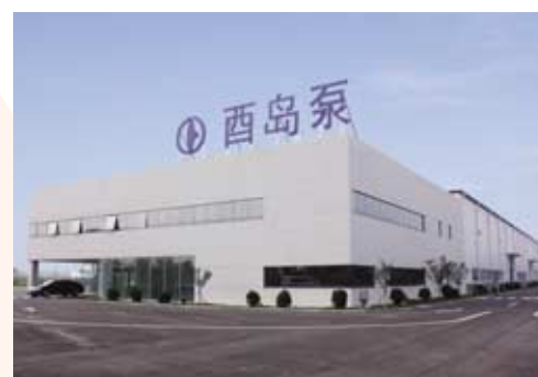
Torishima Pump (Tianjin) Co., Ltd., China
