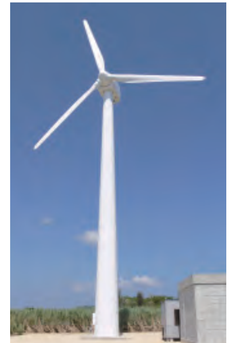
100kW wind turbine
